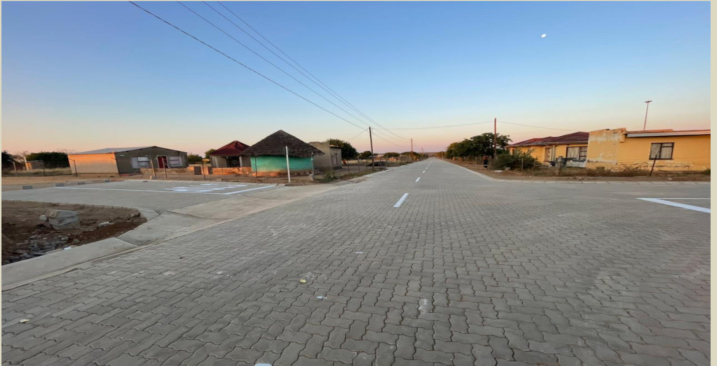
Shawela upgrading from gravel to paving
